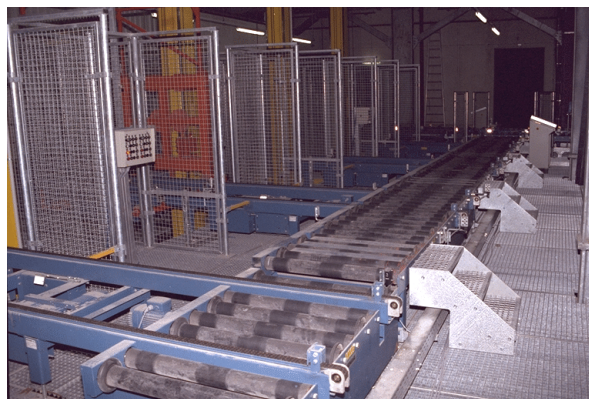
Figure 1.4: One of the circular conveyor belts of the elevator system (courtesy of Herlitz PBS AG).
